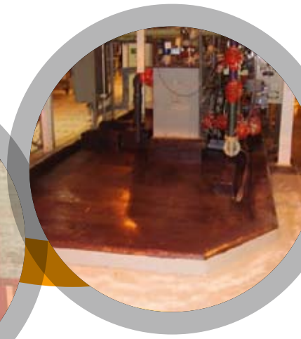
Chemical Storage Areas
